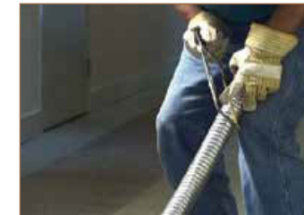
Using hacksaw to cut two adjacent convolutions
