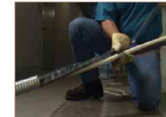
Removing mylar tape from conductors
