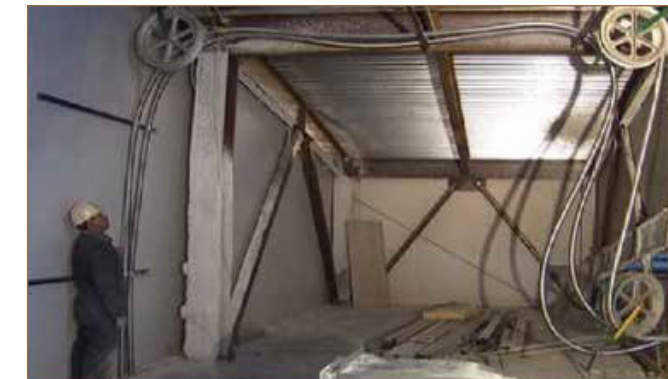
Example of using multiple sheave wheels to achieve required bending radius
