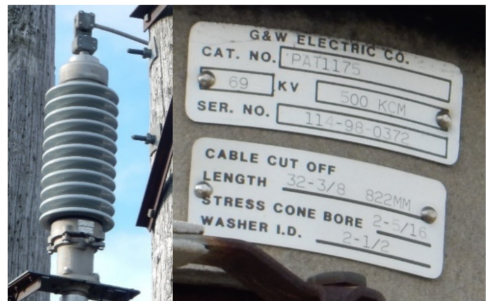
Figure 2: Photograph collected from aerial drone detailing the pole-top termination manufacturer's part numbers and specifications.
