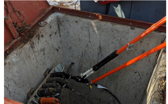
Figure 3: Completing MIC injection in a vault
