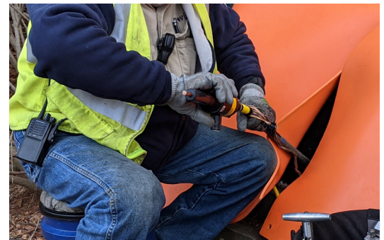
Figure 1: Assembling the MIC body onto the cable.
