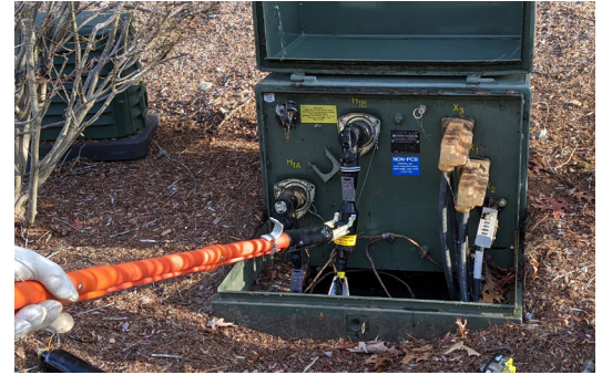
Figure 3: Completing MIC Injection.
